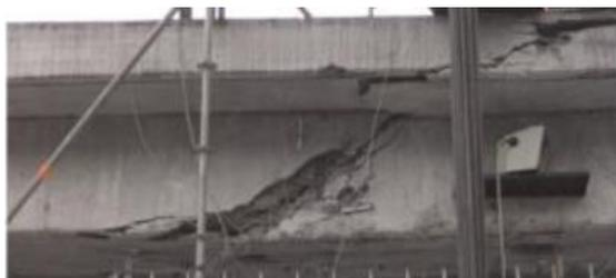
Figure 10. Observed shear failure next to concentrated loads [3]
